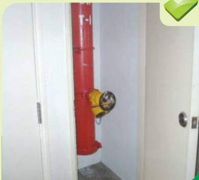
No storage of items within dry/wet riser compartment.
