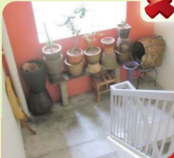
Obstruction to means of escape (staircase).
